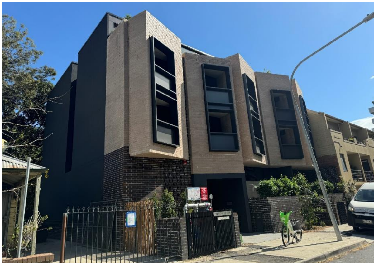
Figure 7: Neighbouring property at 1-3 Goddard Street
