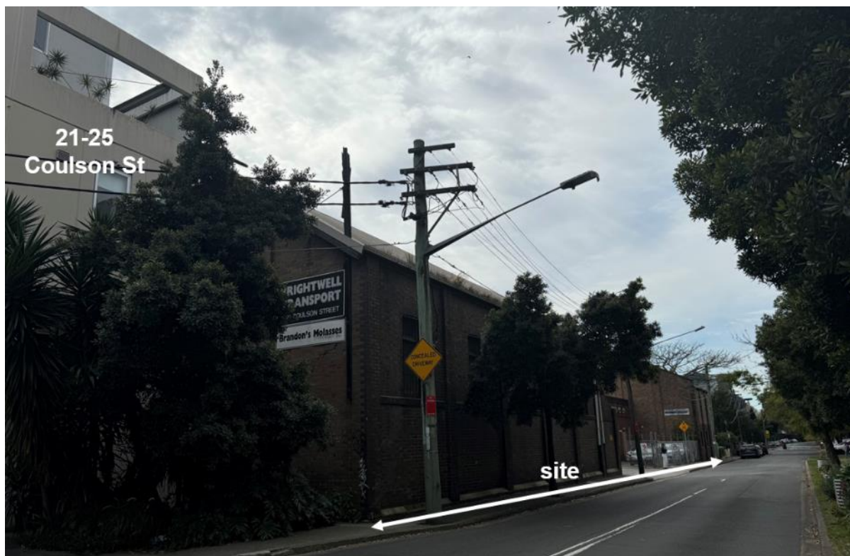
Figure 5: Site (7-19 Coulson Street) viewed from Coulson Street
