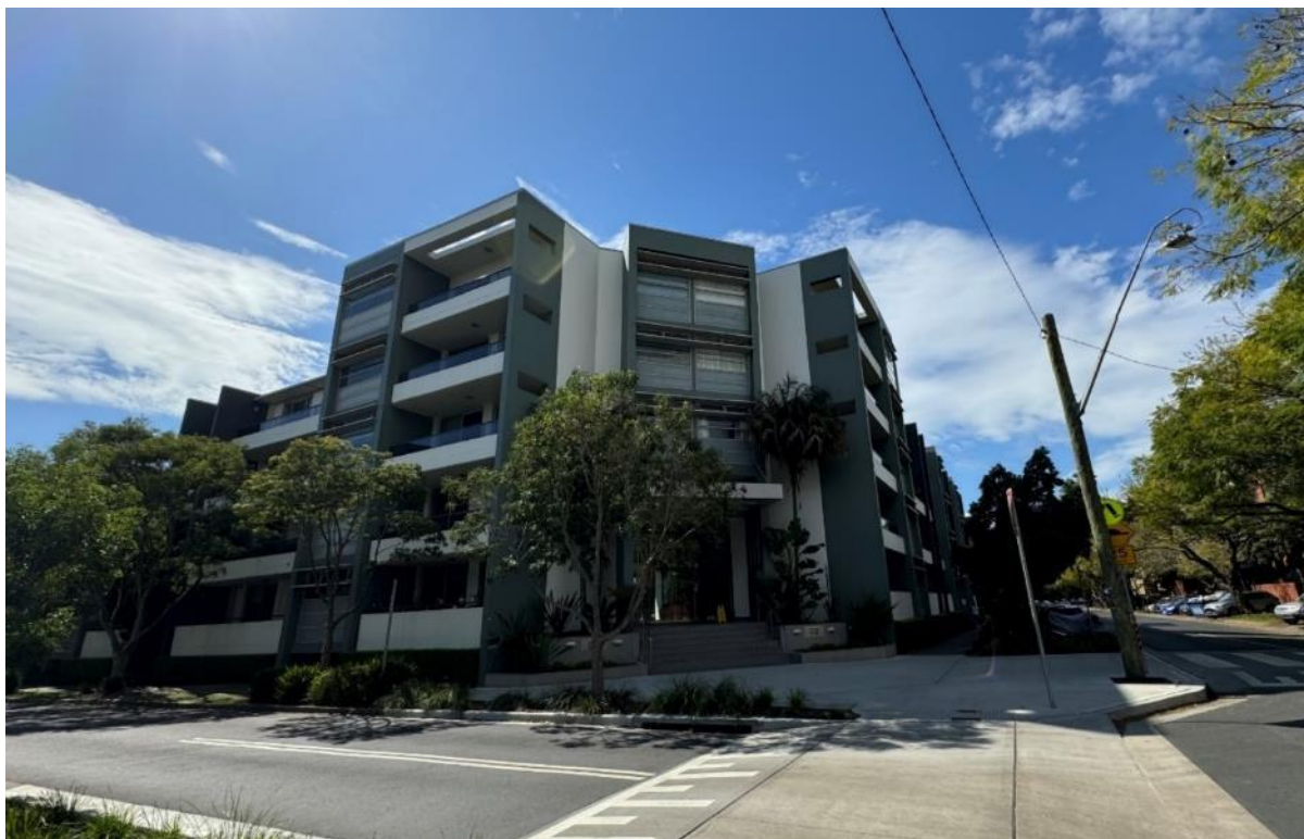
Figure 9: Neighbouring property at 20 Eve Street
